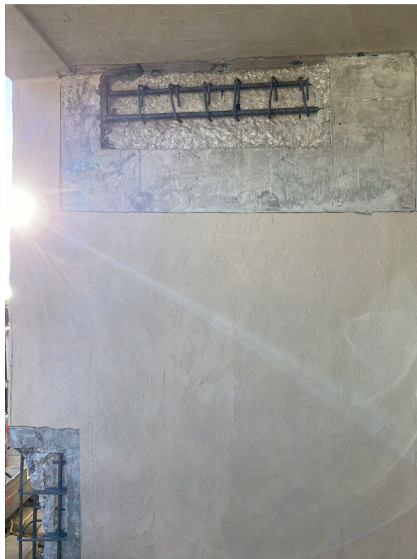
Picture 2: Completed concrete excavations
