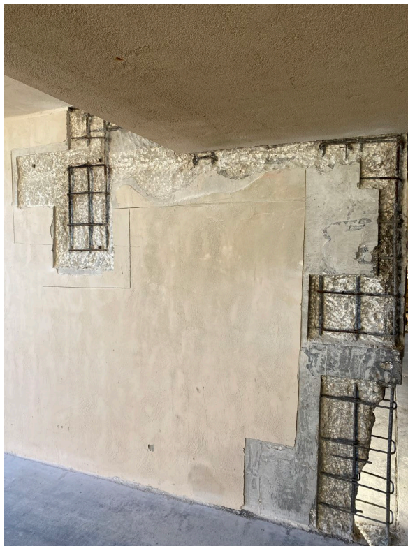
Picture 1: Completed concrete excavations
